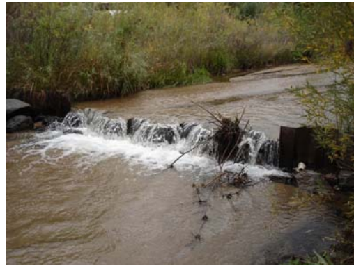
Grade Control Structure along E. Plum Creek
